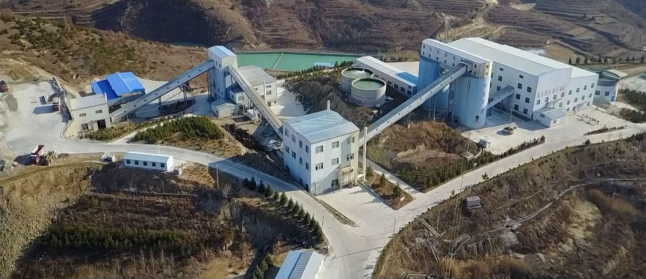
Processing Plant – 6,000 tpd
