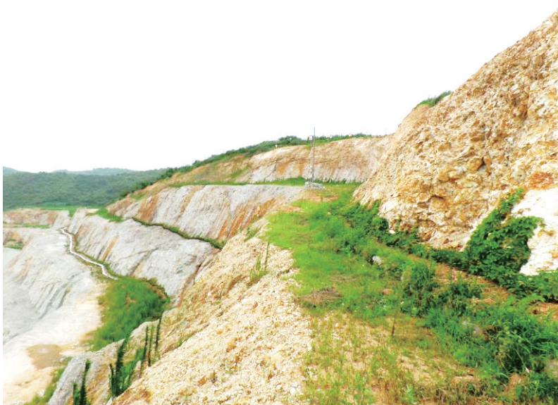
Figure 18-2: Revegetation on the Open Pit Wall of Mining Area
