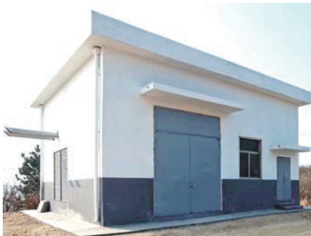
room for diesel generator
