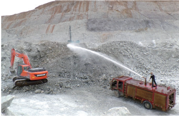
Figure 18-1: On-site Water Sprinkling
