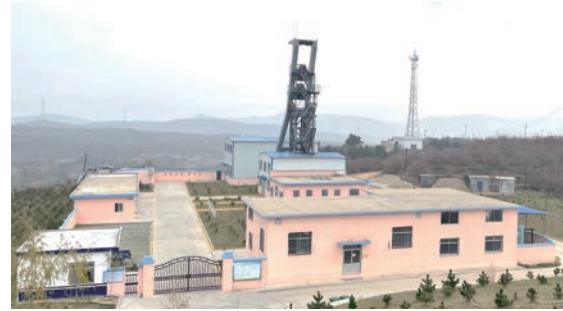
Industrial site of auxiliary shaft
