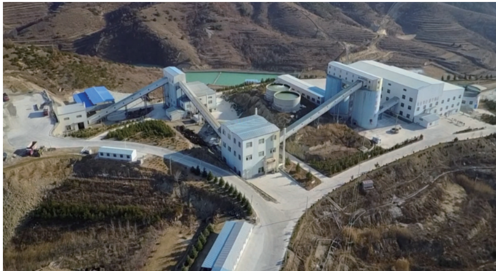
Figure 15-2: Aerial Photo of the Processing Plant
