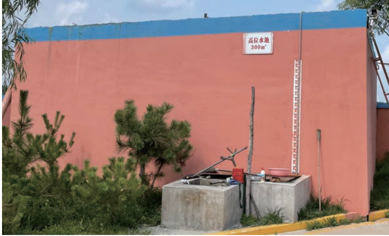
Figure 14-9: Elevated Water Tank
