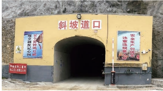
Access ramp's portal
