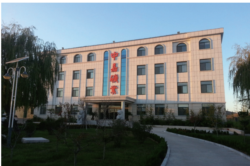
Figure 16-6: Off-site Office Building
