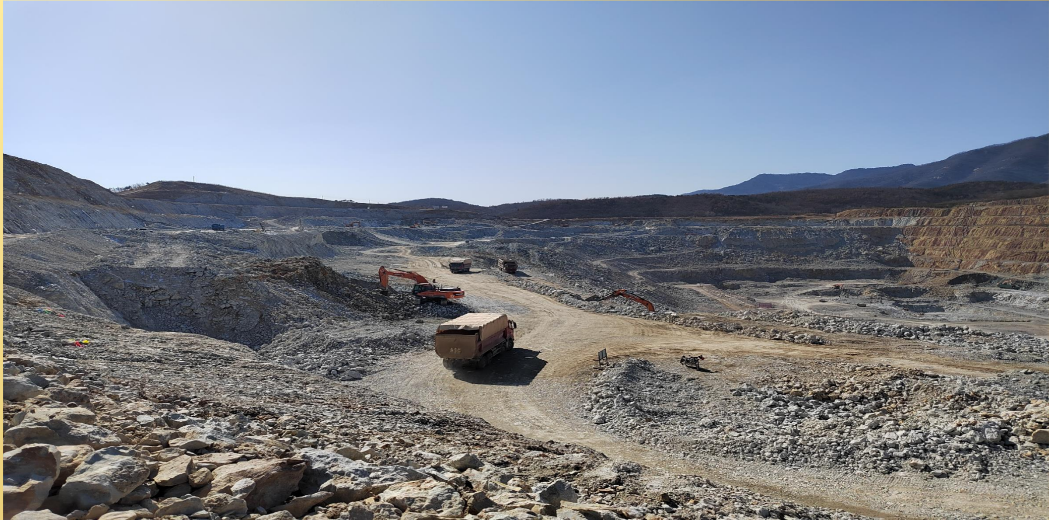
Open-Pit expansion work
