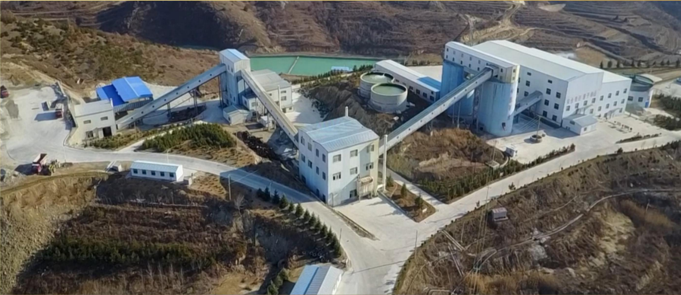
Processing Plant – 6,000 tpd
