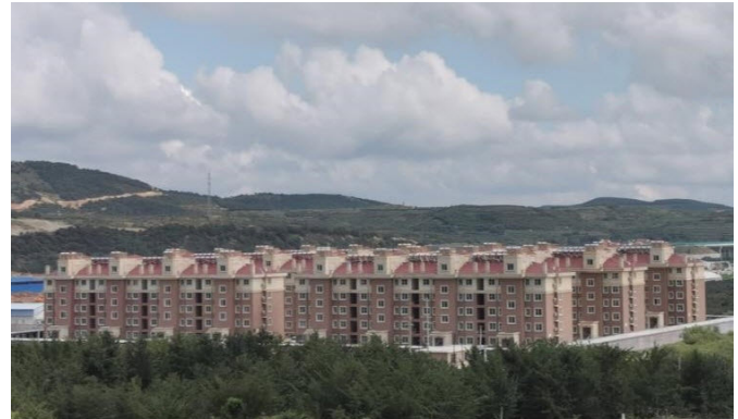
Figure 1: Songjiagou Apartment Complex
