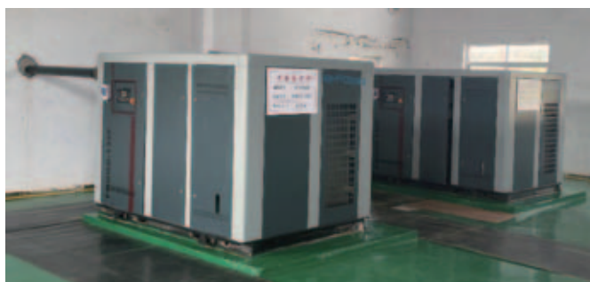
single screw air compressor
