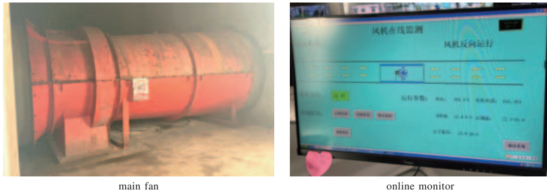
Figure 14-6: Main Fan at the Portal of Upcast
