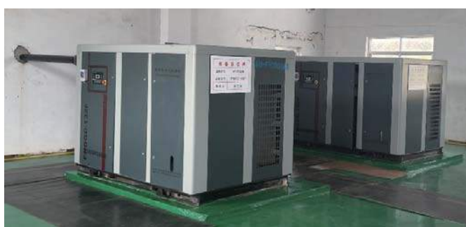
single screw air compressor
